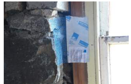
Specialist tapes like this allow for a robust and airtight seal between the window frame and adjacent plaster, but need to be installed first
