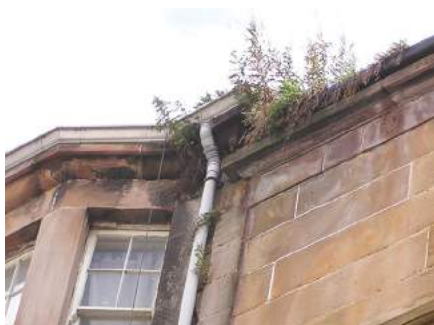
One of the most common problems is of blocked gutters and downpipes
