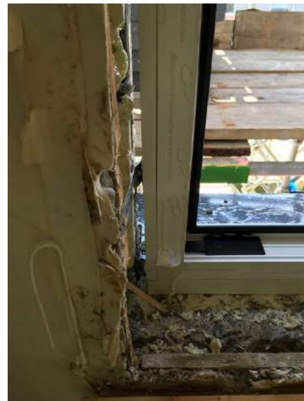
Brand new windows installed but note the gap around the frame which is normally sealed with expanding foam
