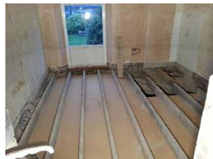
In this renovation, vapour permeable boards were used to contain the insulation, they were taped along all edges before the insulation was installed
