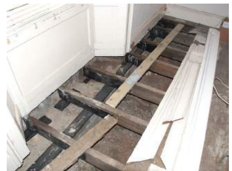
These joists are in reasonable condition but the masonry around is damp, so a sub-floor new vent is required and each joist end has been wrapped
