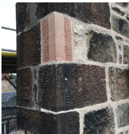
Cement pointing (still visible to the left) has been removed from this stone faced chimney stack and replaced with a lime mix. In addition, a damaged stone has been replaced with a matching natural stone indent.
