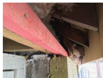
It is important that the roof insulation above meets the EWI below
