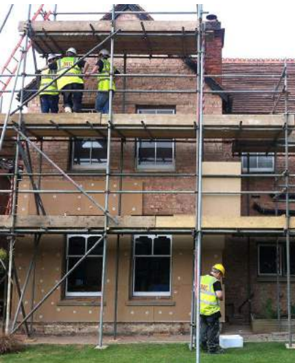
In this project, wood fibre EWI is being installed over a solid brick property © Natural Building Technologies
