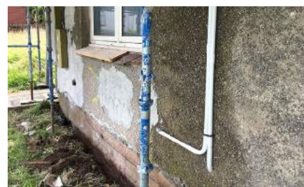
In this project underlying render failures were repaired, conduits installed for all external cables and rainwater and waste pipes re-fixed to allow the insulation to extend behind without breaks
