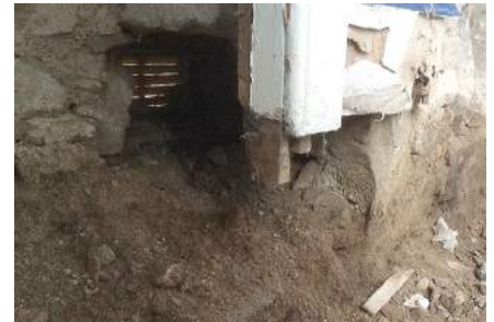
The air vent is above the level of the floor which had become rotten and needed complete replacement. Care was taken to ensure the passage of air was retained to the new solum space.
