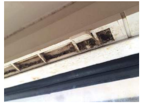
This kitchen trickle vent was completely blocked by debris mixed with grease
