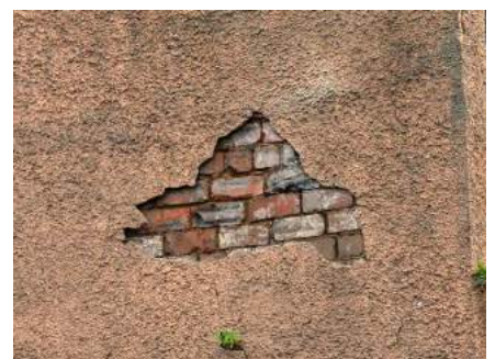
Render fallen from a brick wall. It is likely that adjacent render is 'boss' (loose) and repair is urgently needed
