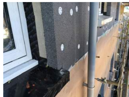
In the same project note airtightness tape (black) is affixed externally to prevent air getting in through the gap
