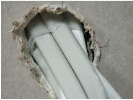
Cables protruding through plasterboard where no service void has been provided meaning the vapour barrier here has been breached
