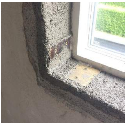
In this example, the reveal has been insulated with a natural, vapour permeable insulating plaster to counteract the poor performance of the thinner walls, and to complement the new windows
