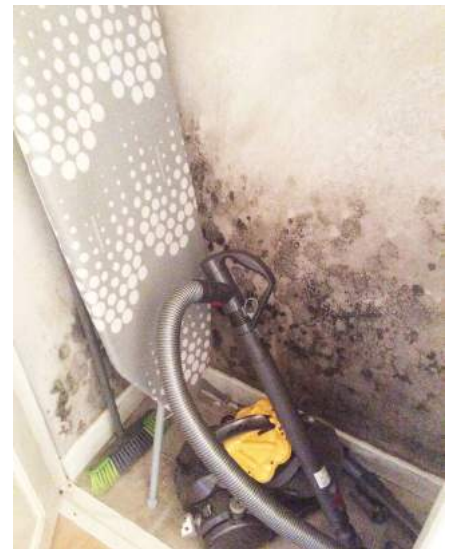
This cupboard developed mould after this flat was retrofitted with external wall insulation. The insulation didn’t extend to the close wall (the cupboard backs onto the close) making this the coldest surface. This unintended consequence creates health risks for occupants and requires additional costs to resolve.
