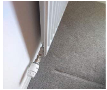
Thermostatic radiator valves, or TRVs, allow each radiator to be individually controlled meaning different rooms can be kept at different temperatures to suit different requirements
