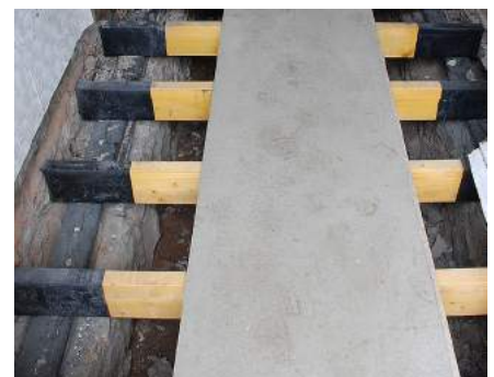
The joists in this hallway were rotten, so new joists have been inserted, with protected ends and sitting on a new DPC
