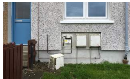
In this project, getting the gas company to move the gas meter boxes proved too difficult and as a result the insulation has been formed around them leaving a significant thermal bridge with a risk of cold surfaces internally and mould
