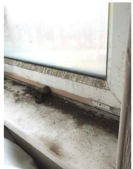
The trickle vent in this bedroom window was kept closed, as was the door, meaning there was not enough fresh air to clear the moisture in the air, leading to condensation and mould on the coldest available surface – the window frame and reveals
