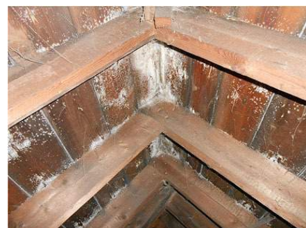
A consequence of warm, moist air entering the loft area but not being adequately ventilated away, hence the importance of ventilation at the eaves
