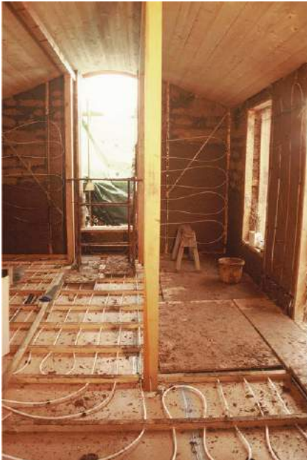
Underfloor and wall heating pipes installed on a small building in the Scottish Borders. Location of the pipes and the use of low level radiant heating pick up on both of the sections on human thermal sensitivity.
