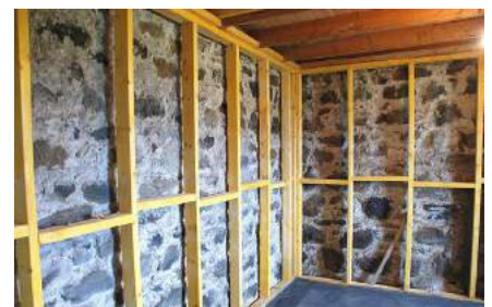
Installing an internal frame, infilled with insulation and a plasterboard finish is relatively simple and inexpensive. In this example, the frame is set apart from the wall to avoid moisture in the stonework affecting the new works.
