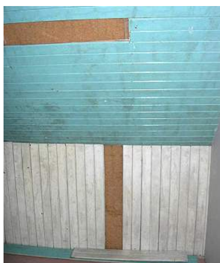
In this attic room, timber linings to the coombe and wall have been removed, wood fibre insulation installed and linings replaced.
