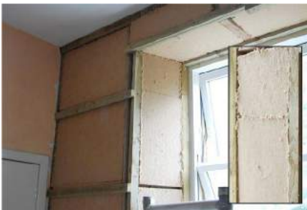
Top image – rigid insulation board installed fairly neatly, but there are still gaps through which heat, air and moisture will flow.
