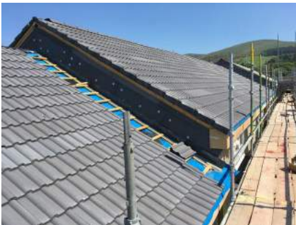
This image shows insulation applied to the upper levels of the gable. This area is often ignored but a small section of the upper flat has been insulated here.
