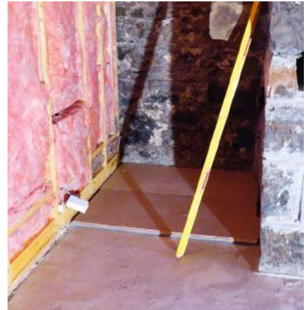
Aerogel blanket bonded to chipboard used as a thin, but high performance insulation over a solid floor. These boards would need to be taped to each other and to the surrounding walls to reduce associated air leakage.
