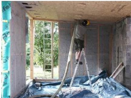
A timber framed 'breathing wall' under construction with hygroscopic recycled cellulose insulation being pumped into ceiling voids and already installed into the walls.
