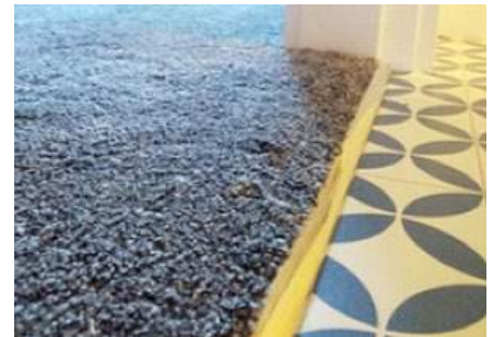
Many planned 10mm clear undercuts are compromised by later carpet installations
