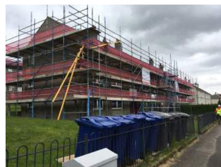
The costs of scaffolding are high, so if it is needed for one works package (e.g. window replacement) it makes sense to take the opportunity, as Renfrewshire Council did here, to also externally insulate and renew the roof finish
