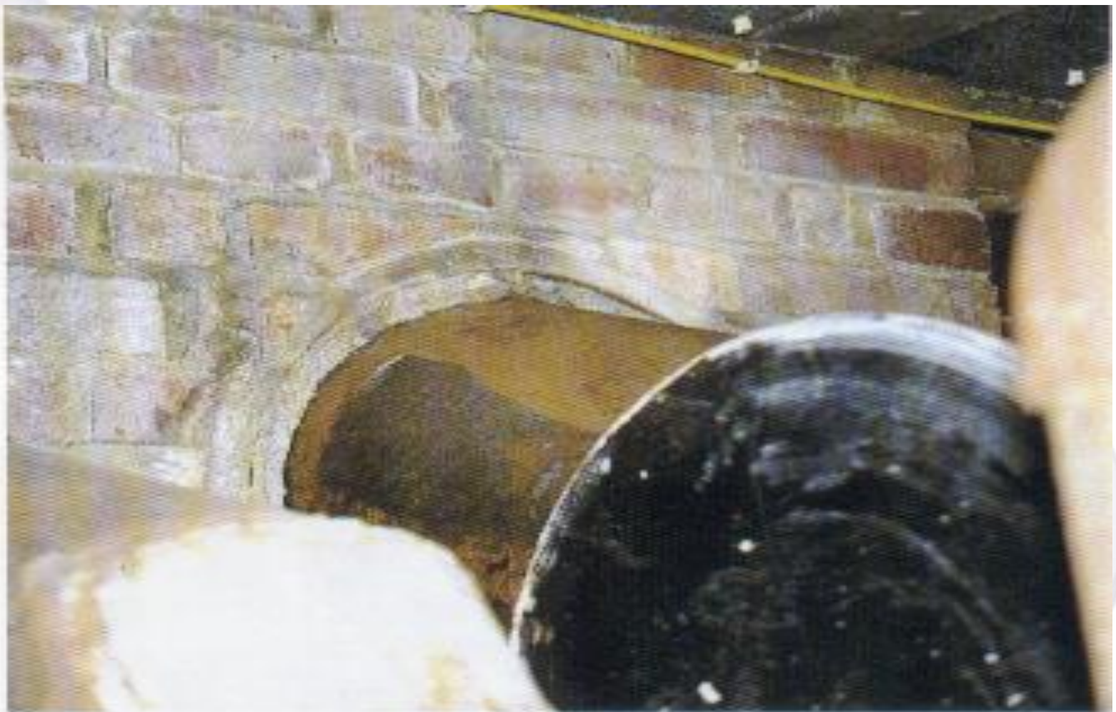
8e Asbestos rope used as packing/seal where pipe passes through a wall.
